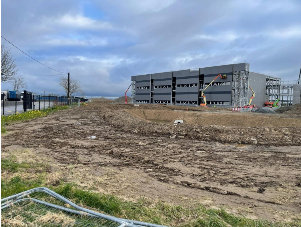
Plate 1: Western area of the site of the proposed amendments to the consented development viewed from the south (photograph dated 31 st March 2026). At the time of writing the area comprises part of the active construction site for a separately consented data centre development at the site
