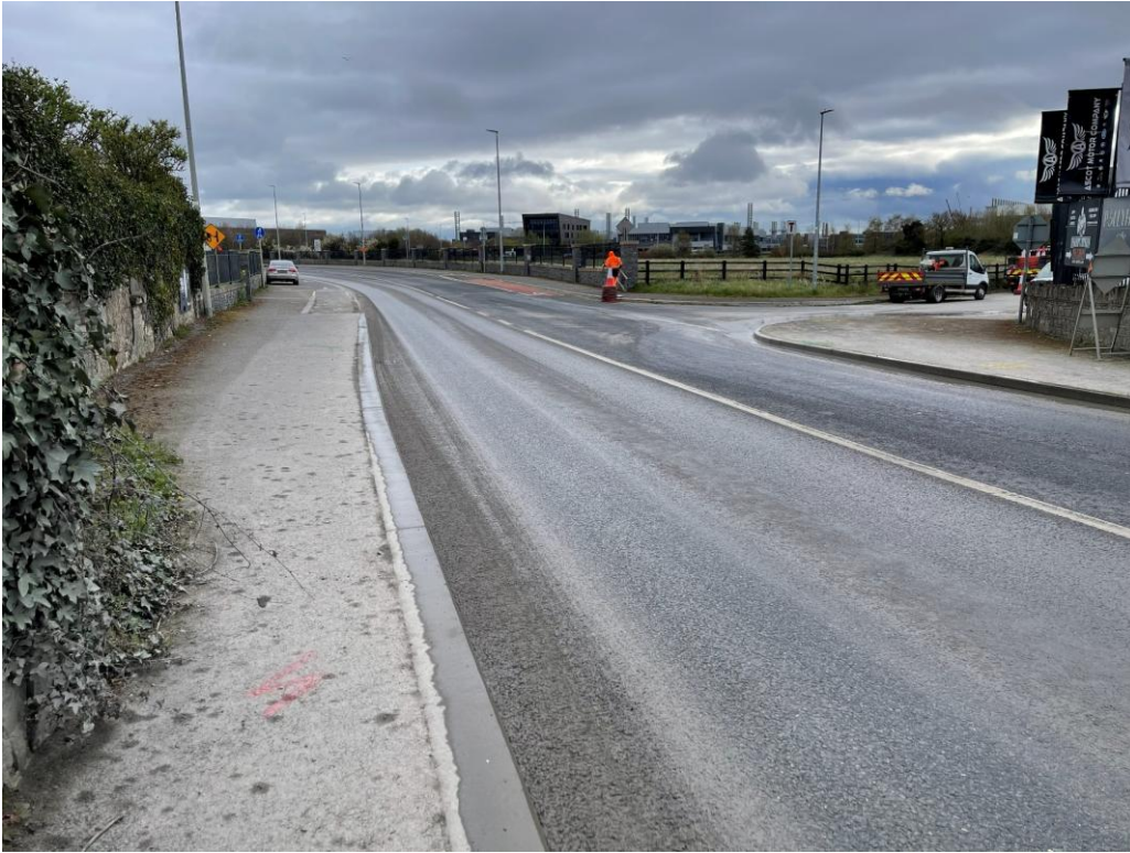
Plate 3: Junction of Peamount Road with the Old Nagor Road, on the route of the transmission lines.
